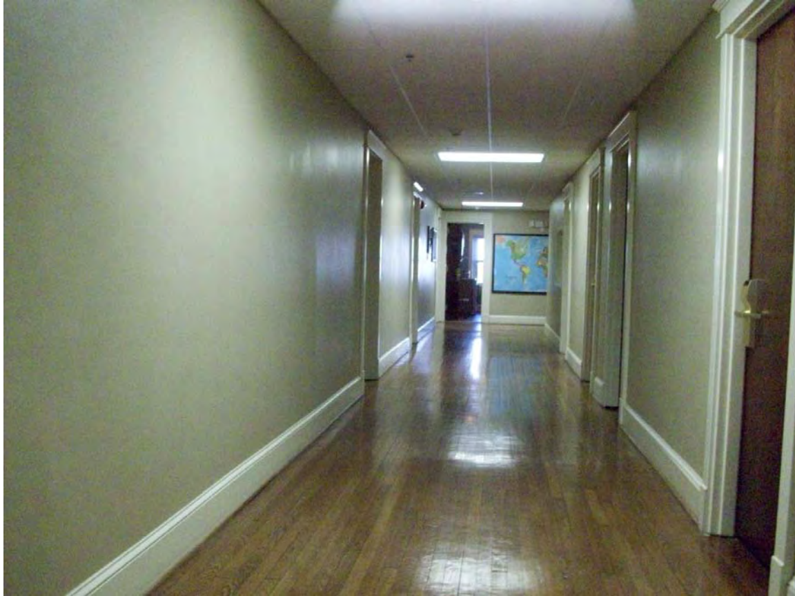
An area damaged by the fire
