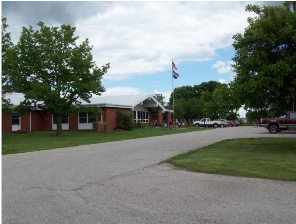
Schuyler County Nursing Home
