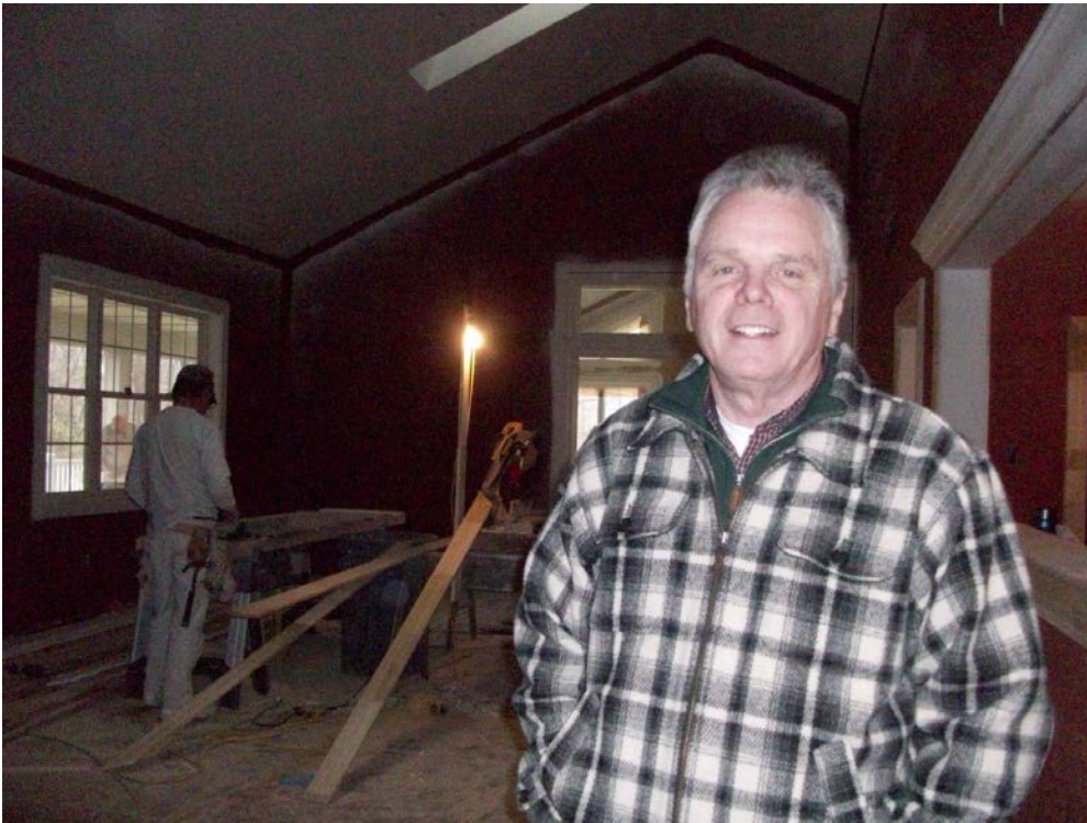
Dolan Residential Care President Tim Dolan overseeing final construction of Les Maisons' next home to open, Lourdes Manor.
