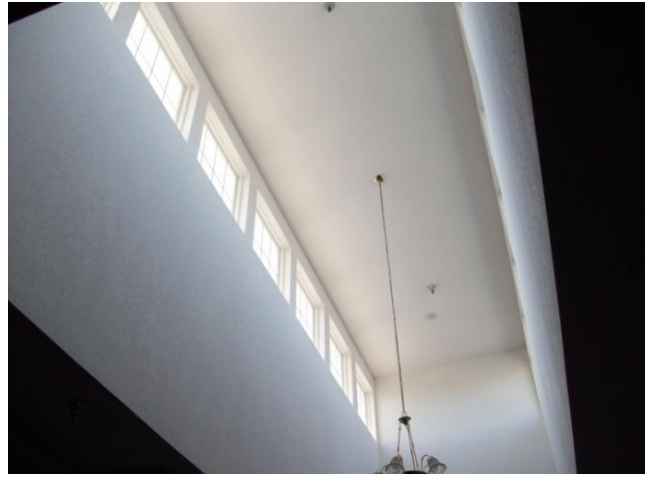
Skylights – Blue River Rehabilitation Center
